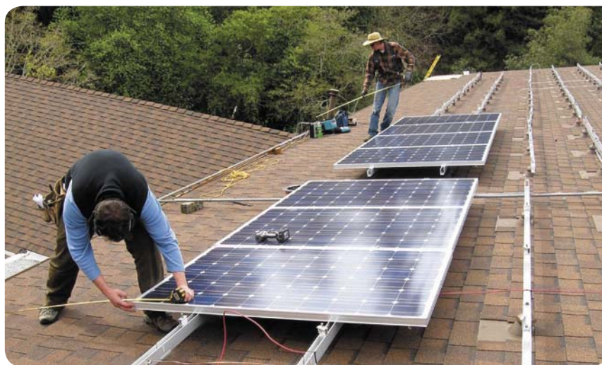
The Lord's work: Workers install part of the 17 kW PV system at the St. John's Episcopal Church in Oakland, California.
